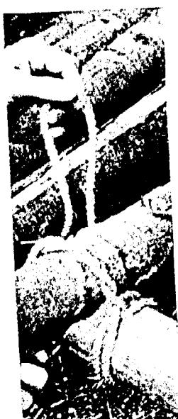
Pull a bight under the stringer and up between the first two spars and slip the bight over the end of the first spar.
