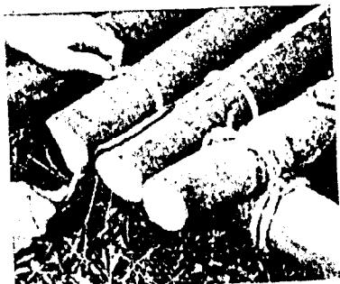
Now pull rope under the stringer and up over the second spar — on the outside of the stringer — then repeat third step.
