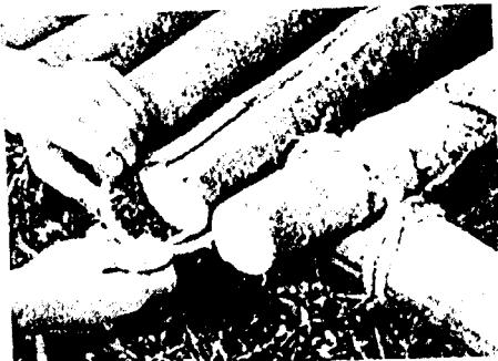
Make a pigtail of the running and standing ends of the rope and pull it snugly over the first spar of the flooring.
