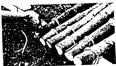
Continue this way until all spars have been laid firmly in place. Finish the lashing with a clove hitch around the stringer.
