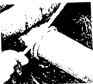
FLOOR LASHING: In floor lashing, start with clove hitch around stringer on which the flooring spars are to be laid.
